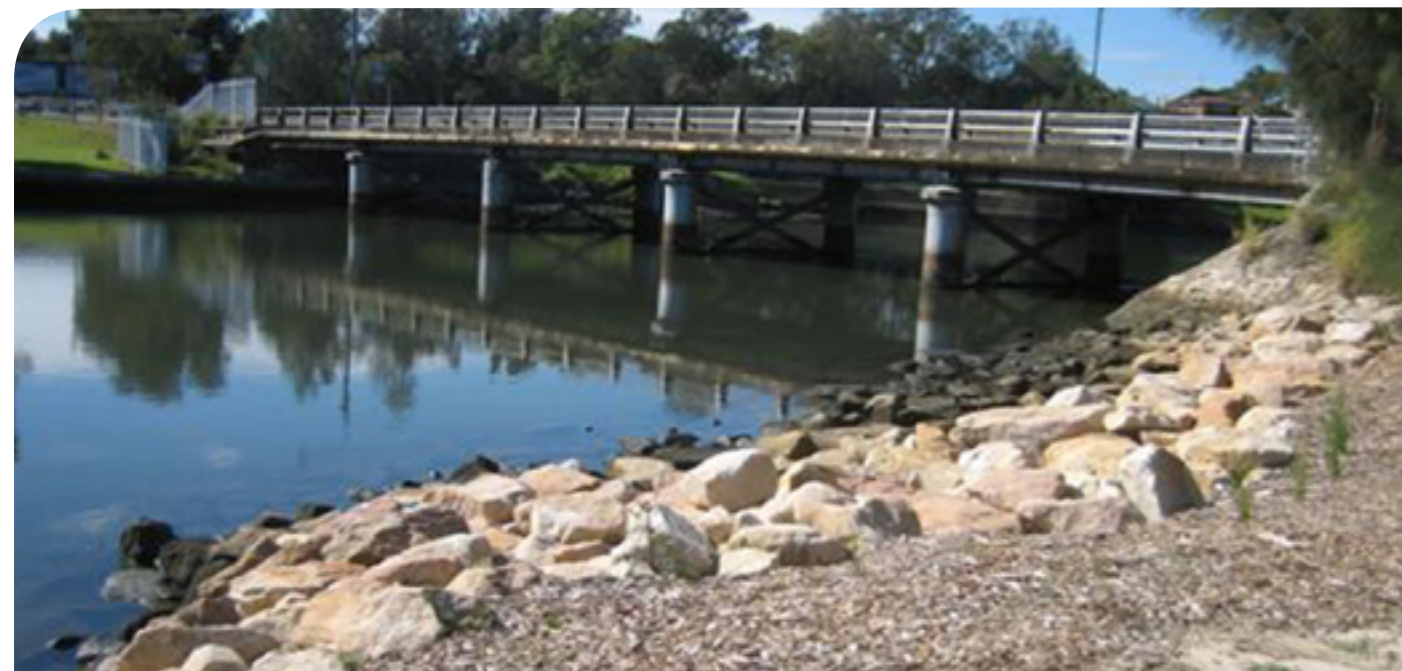
Restoring the Cooks River with bank naturalisation work.
